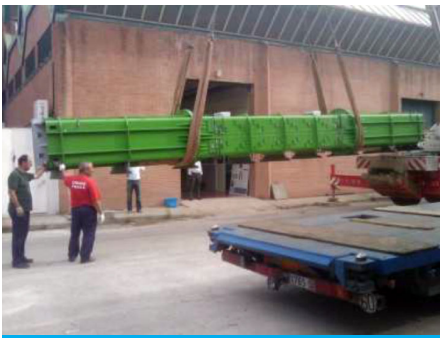
Phase 1 of the base project: Linear machine construction.
